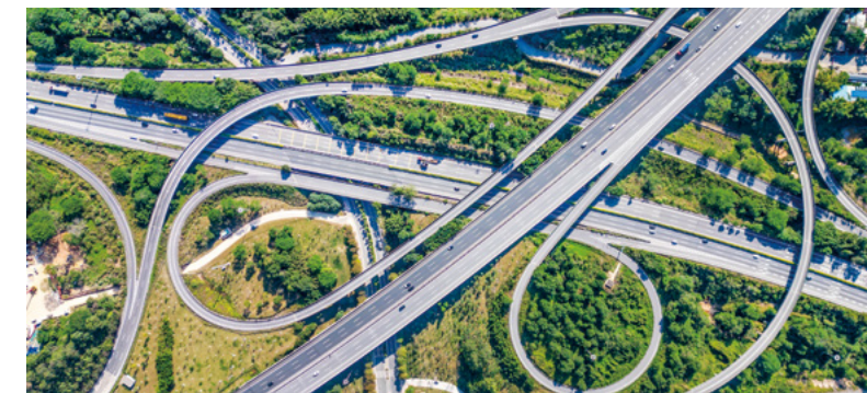
North 2 nd Ring Expressway Reconstruction & Expansion Project
