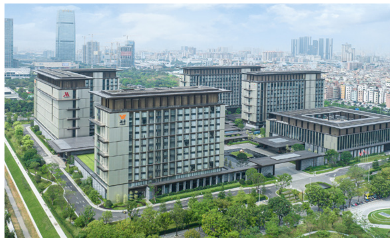
Yuexiu Marriott Complex Hotel Clusters invested by Yuexiu Group in Baiyun District, Guangzhou
