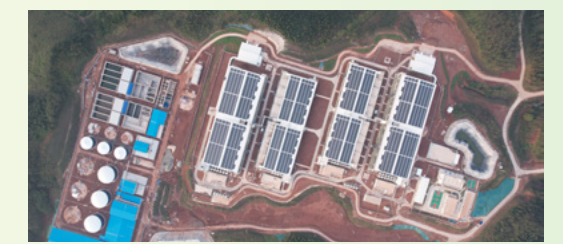
Environmental protection zone of Fengkai Project
