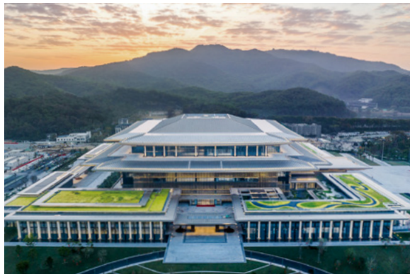
Baiyun International Conference Center Phase II
