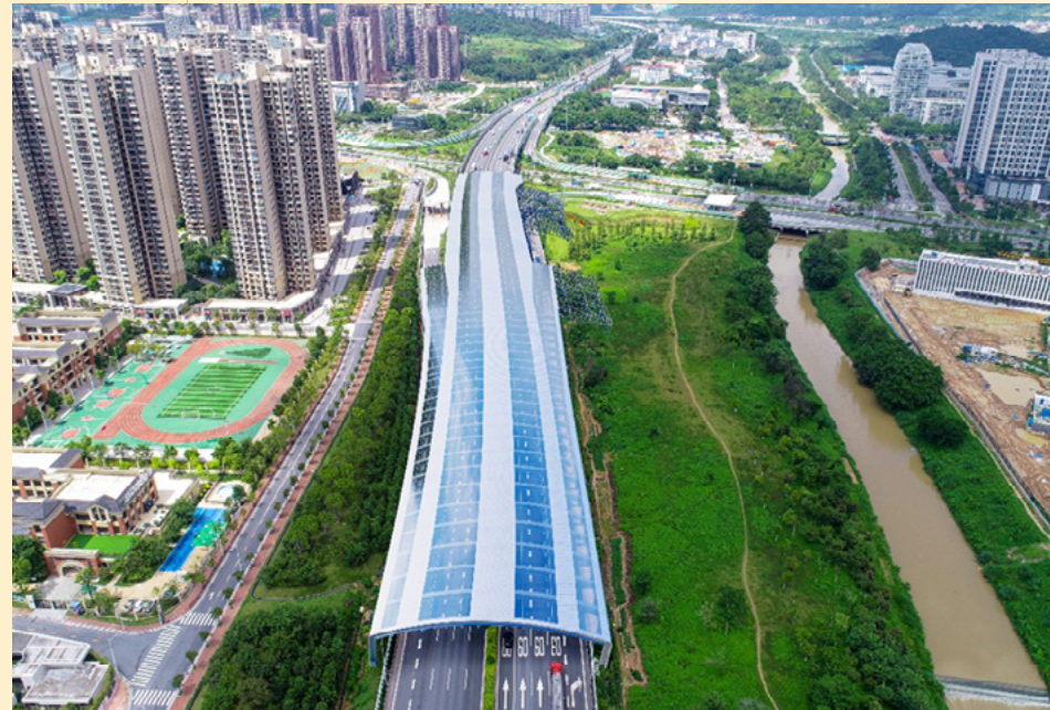
Yuexiu Transport North 2nd Ring Expressway Project
