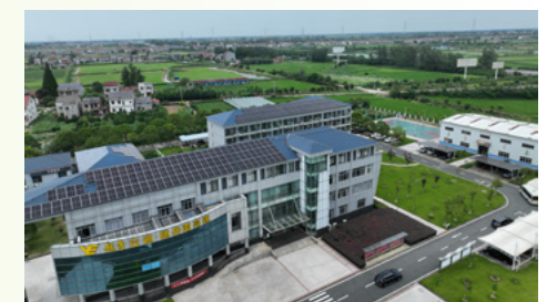
Yuexiu Financial Leasing built a PV project for Suiyuan expressway of Yuexiu Transport
